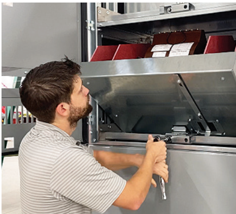
Fig. 3.14. Insertion of Auxillary Modules
