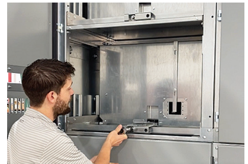
Fig. 3.13. Insertion of Auxiliary Modules
