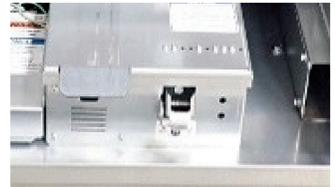
Fig. 1.17. Racking Interlocks
