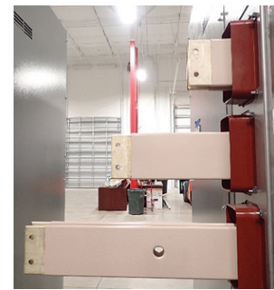
Figure 3.3. Ground Bus
